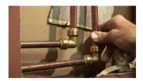
**Copper Type L** ranges from the color of a new penny to dark brown. Copper Type L pipe is also commonly used for general residential plumbing purposes and can be used in outdoor and commercial applications. "Type L" will be printed on the wall in blue and often accompanied by a blue stripe down the length of the pipe.
